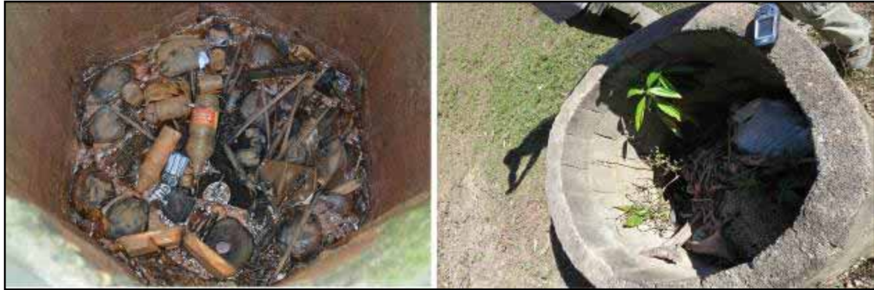
Fig. 44 Abandoned wells filled up with waste, Cowpen.
