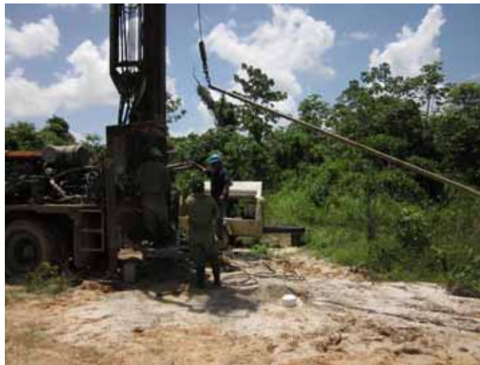
Figure 3: Rural Development crew setting up for hydraulic testing of HGE-1
